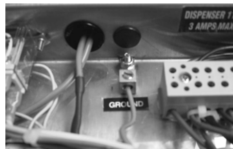
(Ground lug) Figure 2.2.3d
